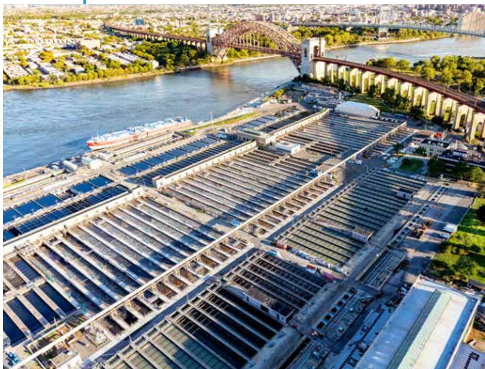
Above: Wards Island Wastewater Treatment Plant in NYC, Randall's Island
